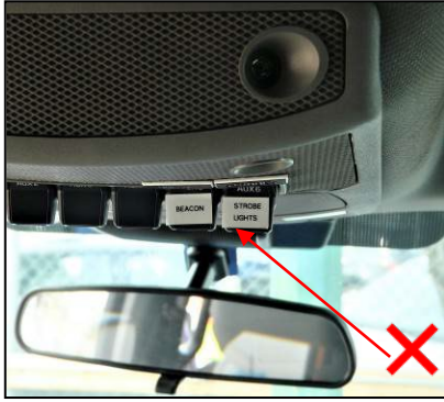
Not Acceptable – Not Permanently Label
